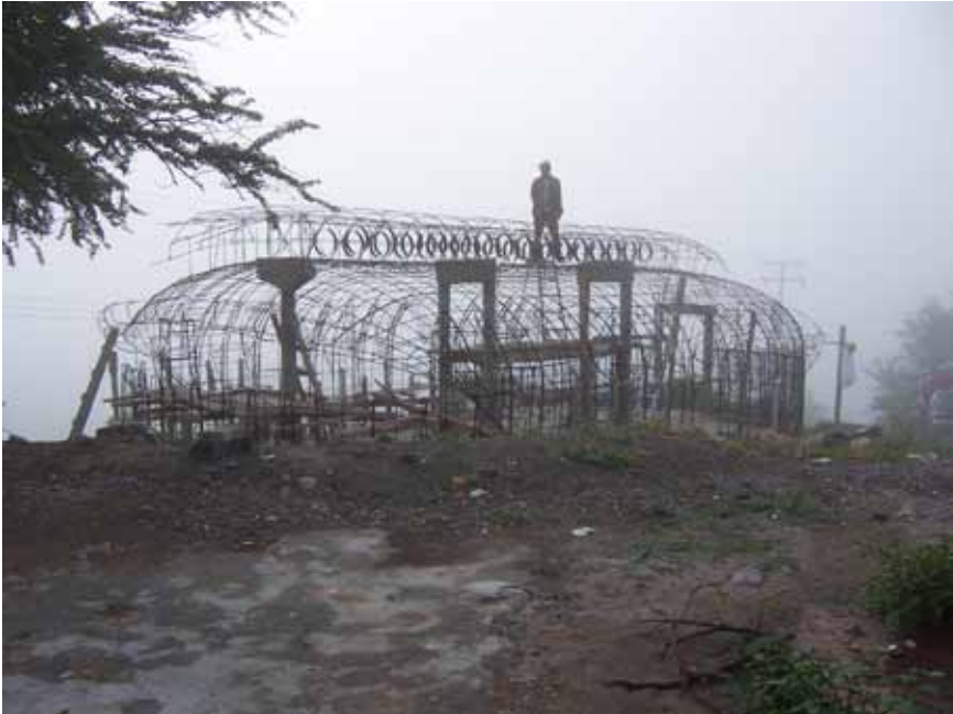
The rebar armature grid rear view
