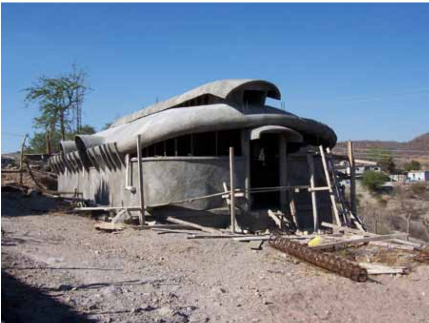
Front of the building with cement coating
