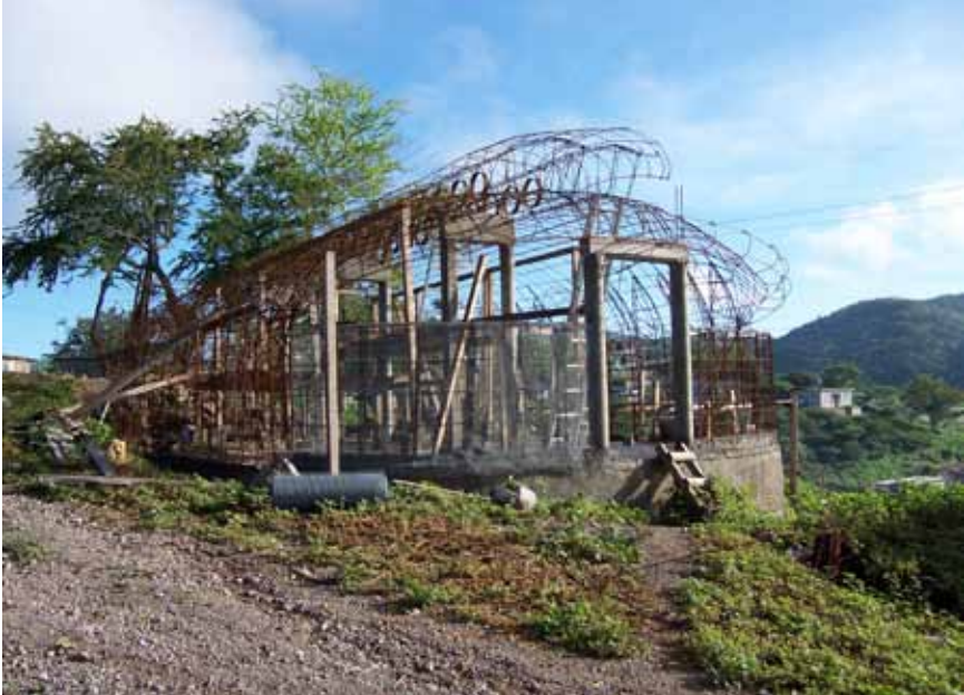
The rebar armature grid front view
